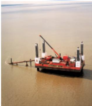
Cables may have to be taken ashore by directional drilling. Hydro Soil Services (HSS) is also an expert in this area. Horizontal directional drilling is an environmentally
