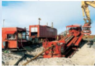
benign, effective solution for installing cables, pipelines and other services in port, river, airport and offshore contexts. It permits traffic to continue without disruption. HSS specialises in two advanced fields of directional drilling: long-distance and large-diameter. During the construction of offshore windfarms these techniques may be applied from the shore-side, or from a jack-up platform offshore for cable landing. Modular equipment facilitates rapid deployment anywhere in the world.
